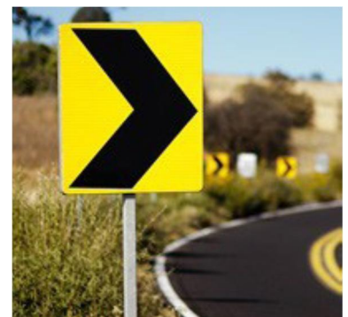
Example Proven Safety Strategy: Chevron Curve Warning
